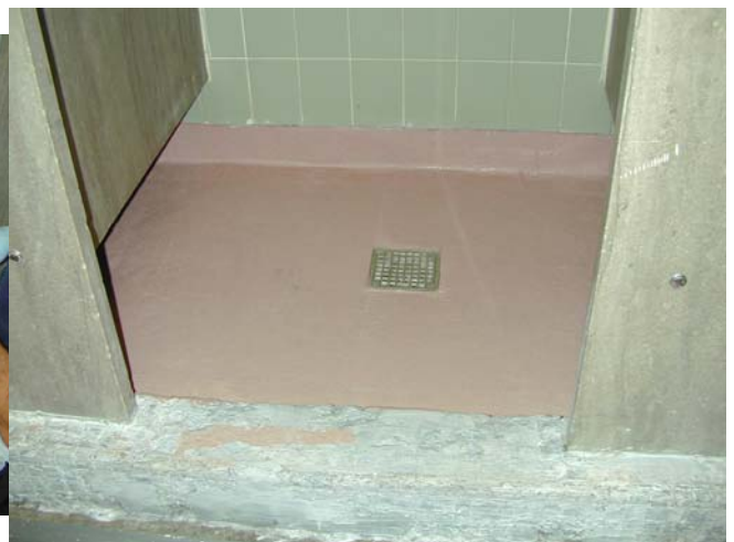
FINISHED MEMBRANE IN SHOWER
