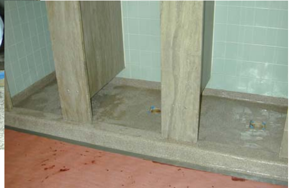
FIRST GROUT SETTLING INTO MATRIX
