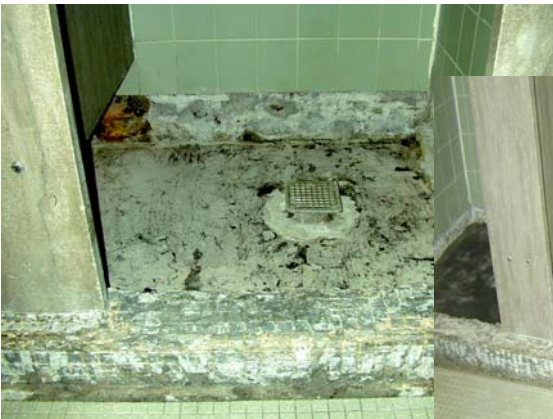
REMOVED SETTING BED
