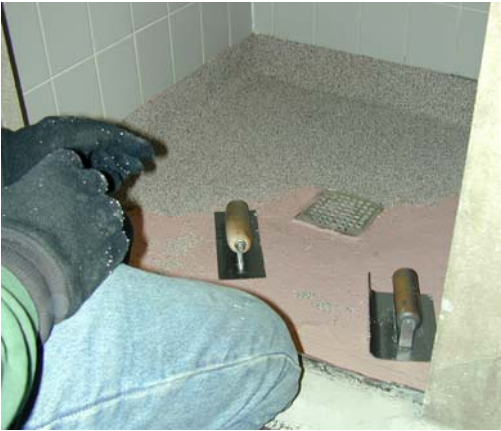
EPOXY APPLICATION OVER MEMBRANE
