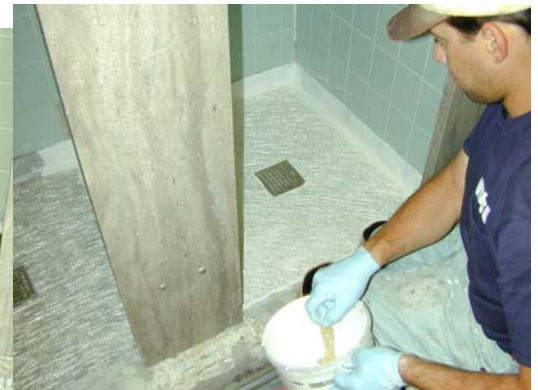
FIBERGLASS REINFORCED WATERPROOF MEMBRANE
